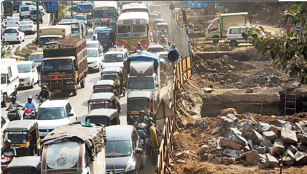
Figure 8: Western express highway excavated for Mumbai metro layout
