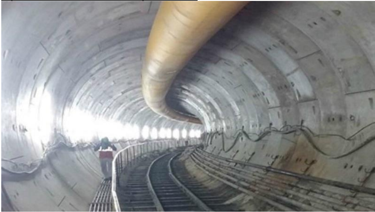
Figure 4: East west corridor underground tunnel
